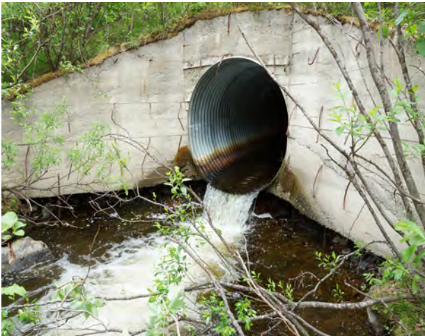
Figure 7. Vuohppejohka before the restoration (main road).
