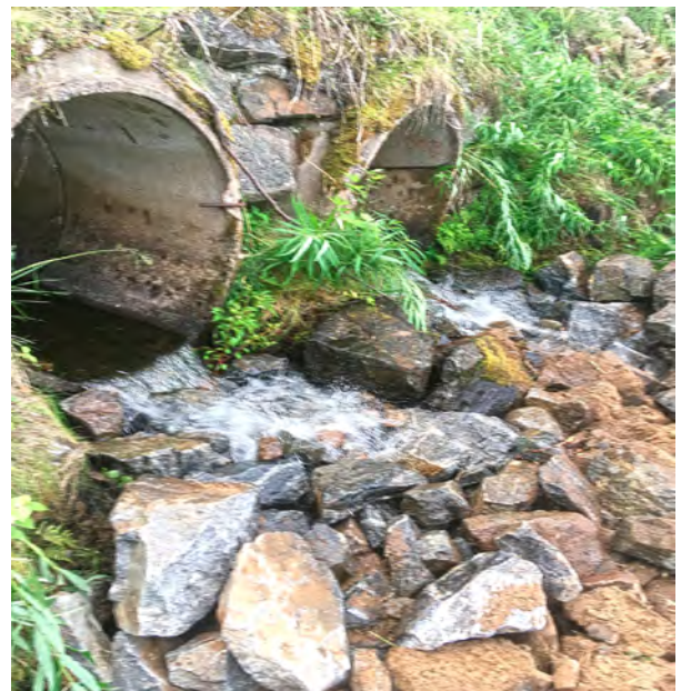
Figure 3. Vuolit Boratbokcájohka after restoration.
