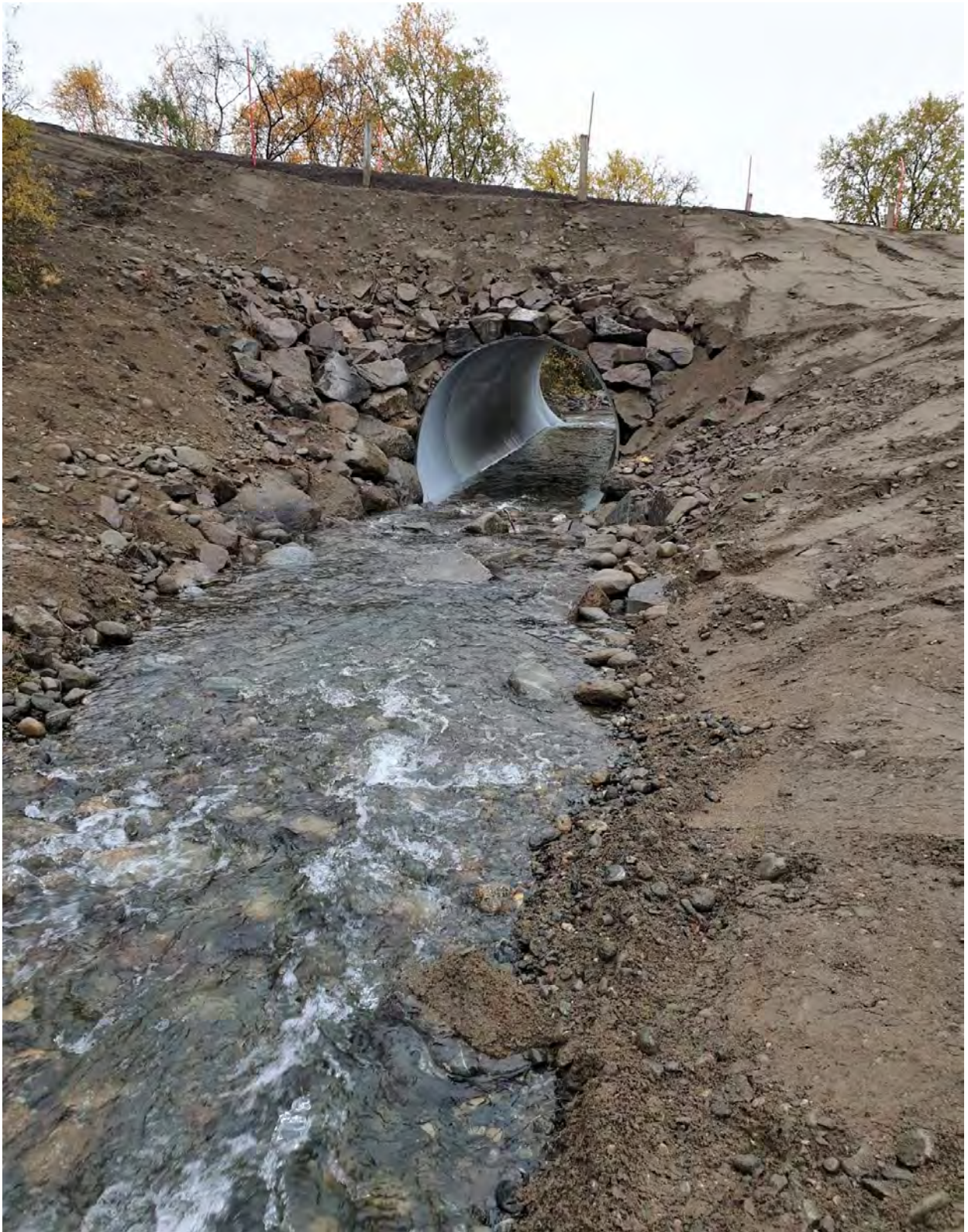
Figure 11. Lišmmajohka after the restoration (Photo: NVE nord).
