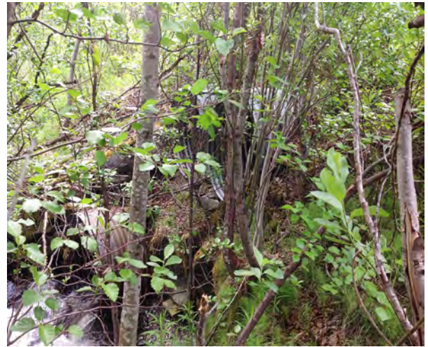
Figure 5. Culverts on the private road at Vuohppejohka.
