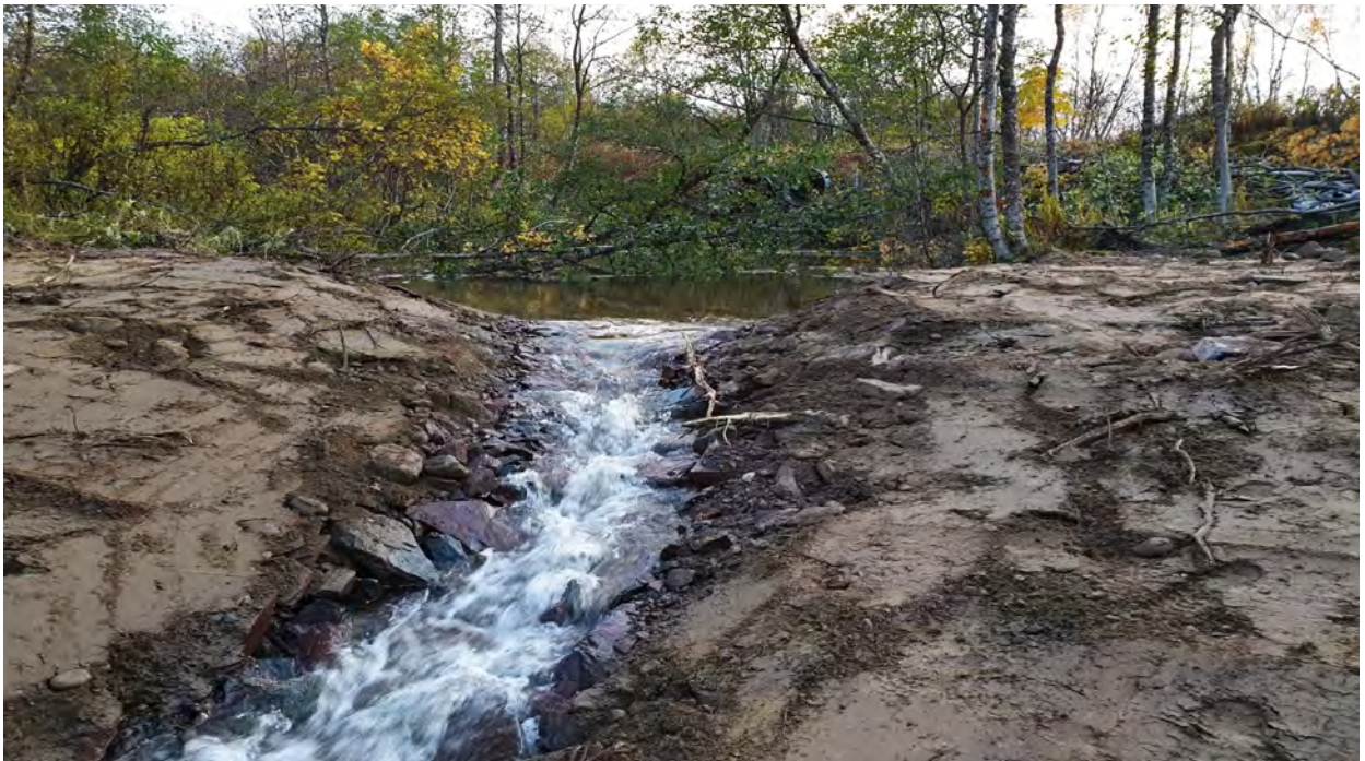
Figure 6. The threshold built to increase the water level Vuohppejohka (private road).
